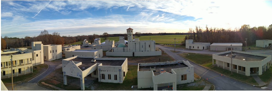
Figure 24. Rooftop view of Cassidy CACTF in Ft. Campbell, TN.
