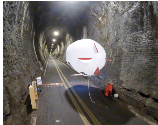
(b) Abandoned railway tunnel in Houli.
