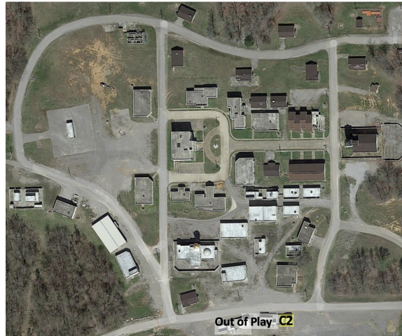
Figure 8. The Fort Campbell Cassidy CACTF, the site of FX-6. The yellow area is the C2 building.
