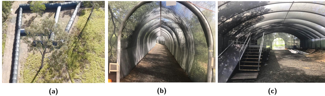
Figure 17. An aerial view of the shade-cloth tunnel with an overall length of over 300 m built at CSIRO's QCAT site in Pullenvale, QLD, Australia (a), an inside view (b) and stairs and mezzanines built inside the tunnel (c).
